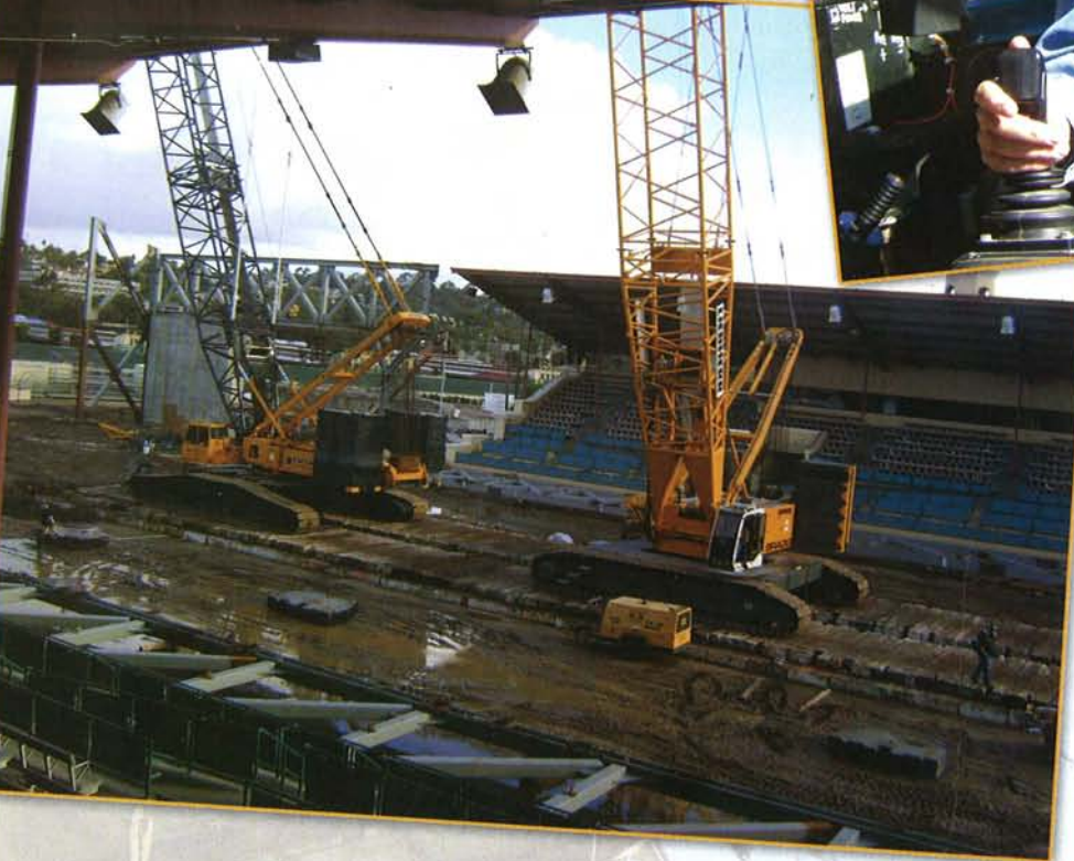
(Left) Liebherr cranes working on the in-field of the Del Mar Thoroughbred Club track.
