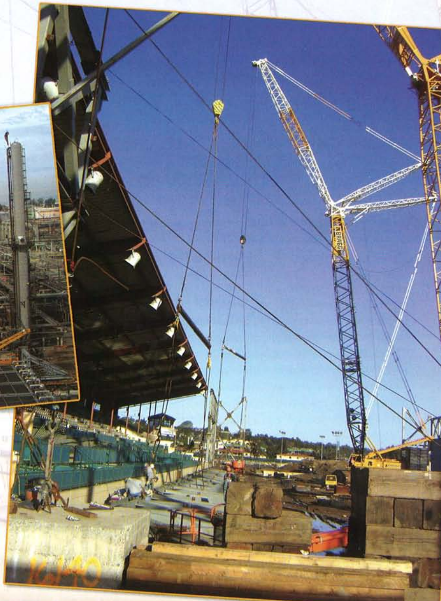
(Right) Bragg Crane Service supplied a Liebherr LR 1300 330-ton crawler crane and a LR 1400 450-ton crawler crane to set the structural steel trusses for the arena.
